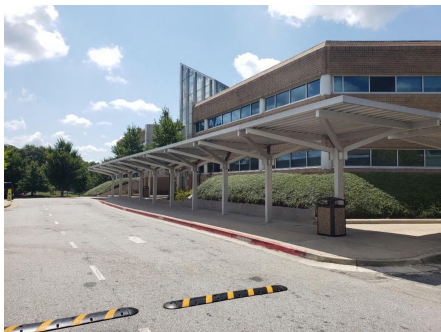
2). Northeast Elevation - Oct 06, 2019
