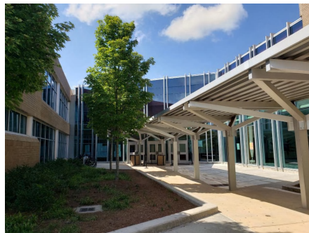
3). Northeast Elevation - Oct 06, 2019
